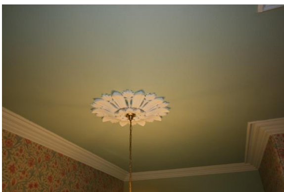
First Floor Landing Centre Rose
